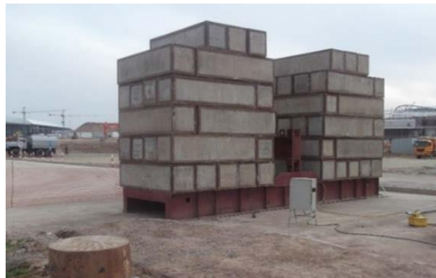
Fig. 2. Static load test on construction site.
