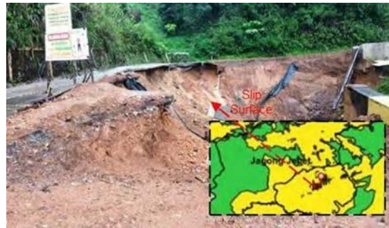
Fig. 3. Verification based on satellite imagery – Slip surface in Jagong Jeget sub-district.
